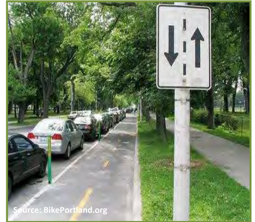
Cycle track installed inside the parking lane in Montreal, Quebec
