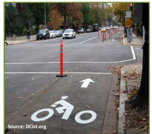
Contraflow bike lane installed on 15 th Street in Washington D.C.
