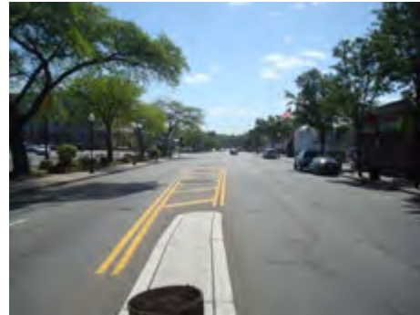
Morris Street, looking east towards Lafayette Avenue
