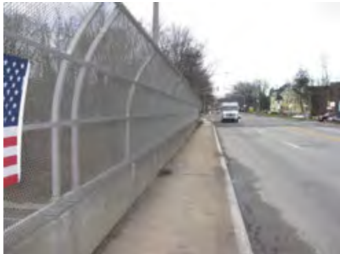
Sidewalk located on Madison Avenue Bridge
